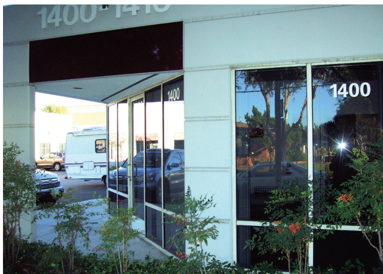
ACA WSO distribution center office in Signal Hill, California.
